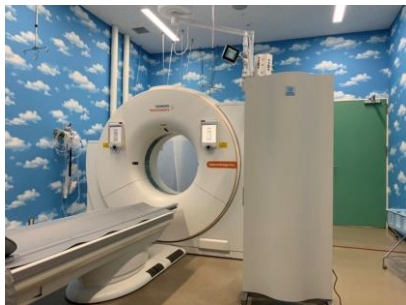
Figure 2: Genano 5250A air purifier in CT room
